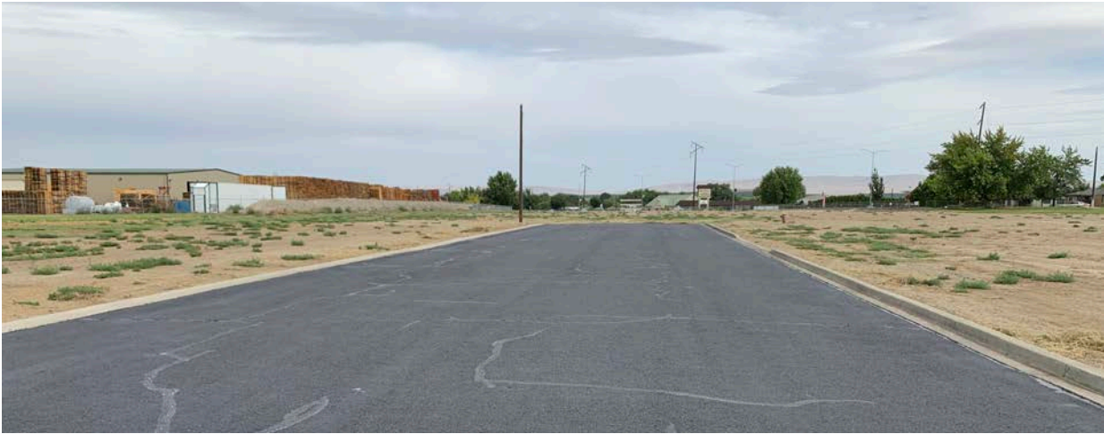
Looking N along access road
